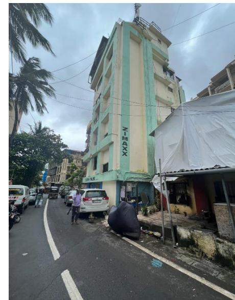
Approach Road and Side Elevation of Zicom House, Bandra West, Mumbai
