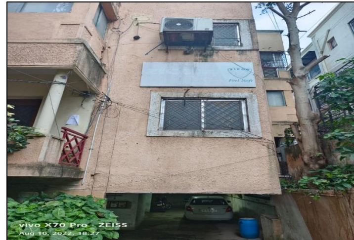
Albert Court, Albert Street, Richmond Town, Bengaluru
